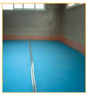
5- Make a mortar slab of about 5 cm. It will be armed or not depending on the mortar type and the direction of the work criteria.
